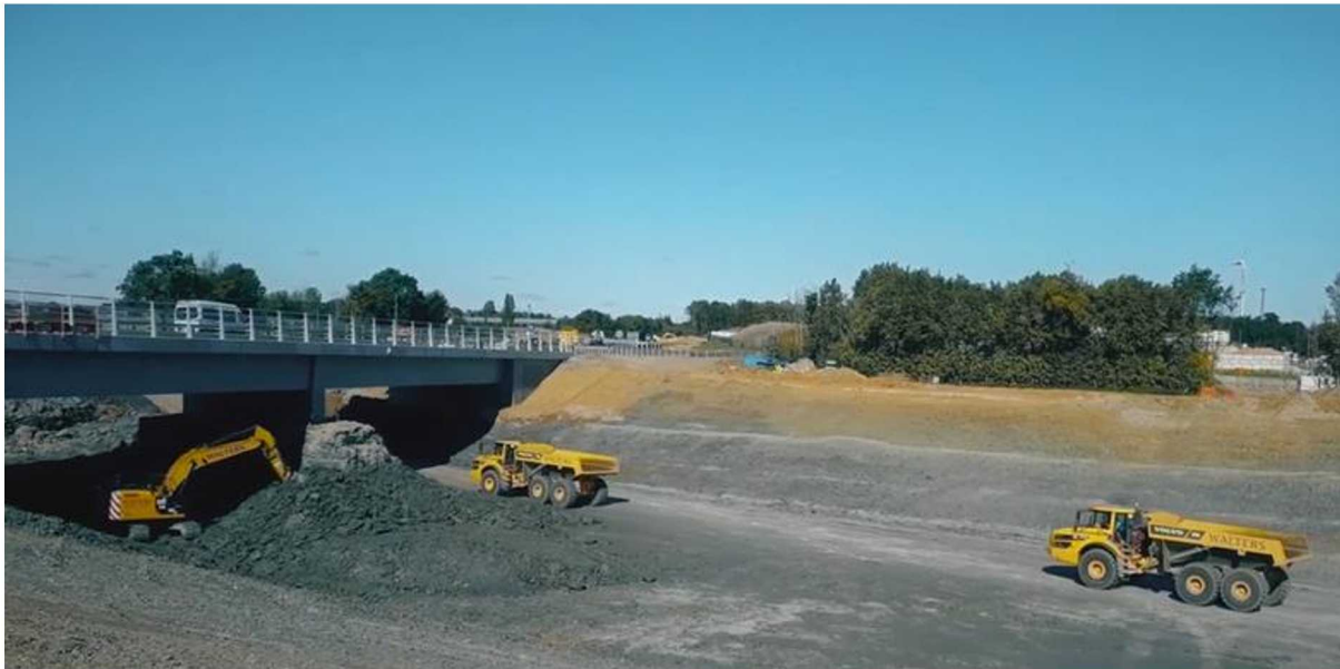
The New Ermine Street Bridge
